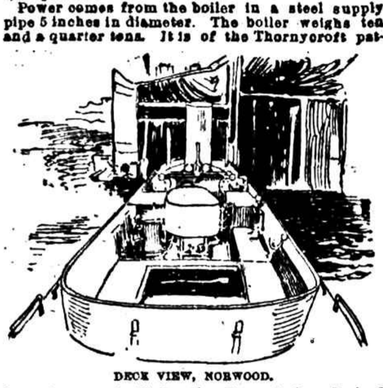
DECK VIEW, NORWOOD.
