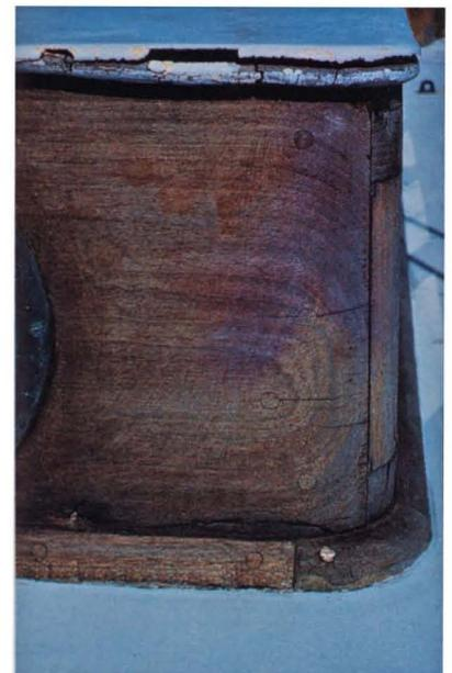
**3. No hidden problems here.** Before the next season begins, the owner knows precisely what will be necessary to bring the joinery and brightwork up to snuff. The tongue-in-groove coach roof planking may need some scraping, but otherwise some minor repairs, a bit of sanding and the traditional seven coats of varnish will suffice. The owner should make it a point to align the slots in the portlight mounting screws.
