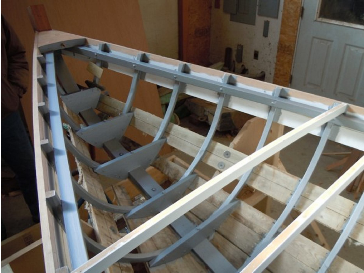
The bow, ready for the remaining deck beams.
