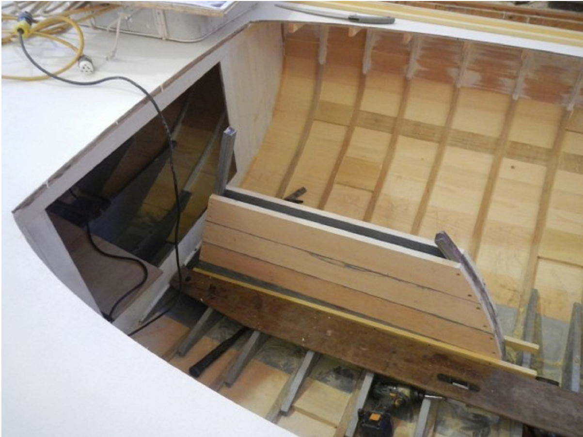
The new centerboard trunk is now almost complete.
