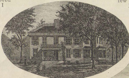
BOSWORTH HOUSE Bristol's Oldest, 1680
