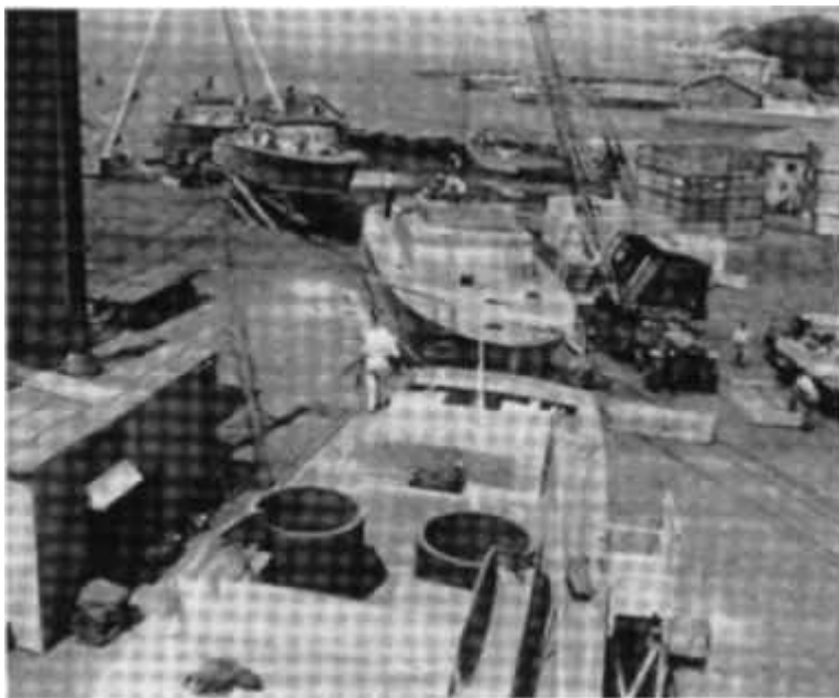
A production line of Air-Sea Rescue boats at the Lower Yard, Walker's Cove - 1944. Eight 85' Army Rescue vessels and thirty-six 63' Army / Navy Rescue vessels were built here. A truck crane is installing Hall-Scott engines. In the upper left background is the tripod designed by Sidney Herreshoff, used to install 10 ton APc engines.
