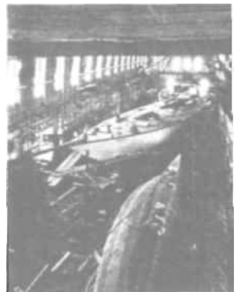
New York 40's Marilee #955 and Rugosa II #983 under construction at the Herreshoff Manufacturing Company
